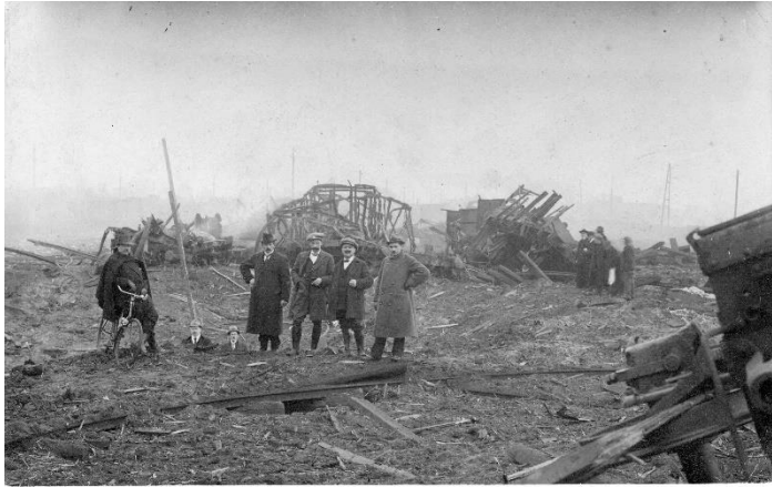
Station Hamont na de enorme ontploffing
